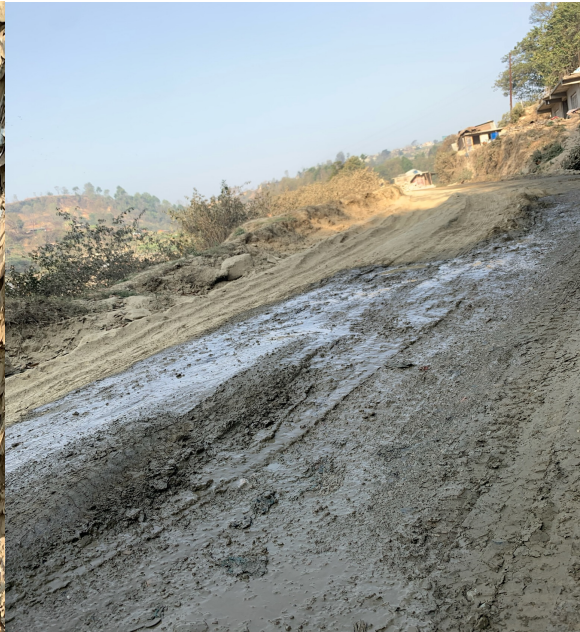
Figure 22 Road between KMC and SLS (©TB)
