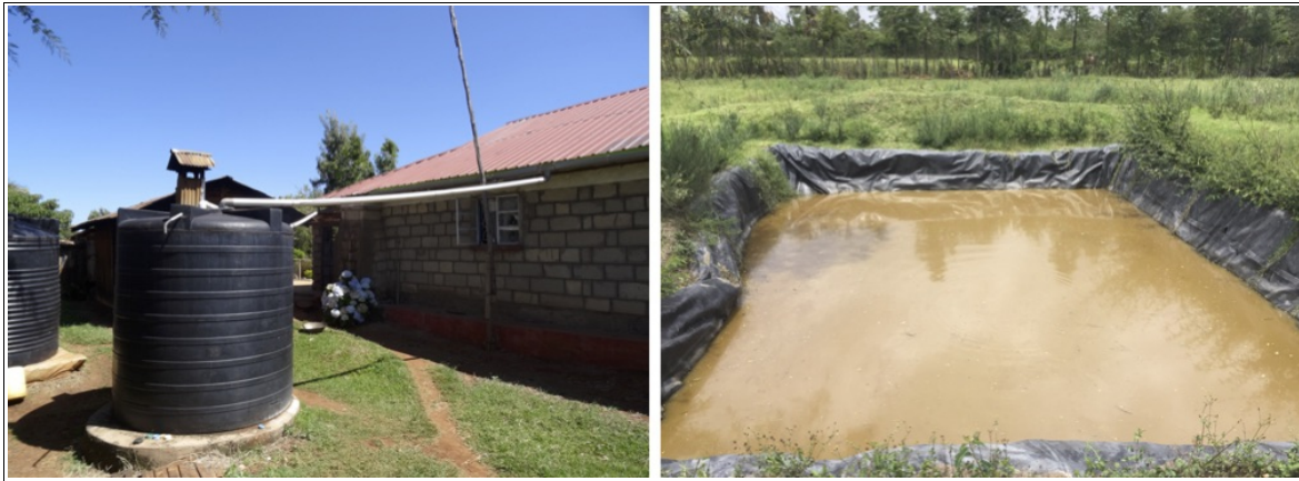
Figure 5.7: Two water harvesting techniques. Left: rain water collection from the roof top, stored in a water tank, left: a water pan dug on the field Pictures taken by the author
