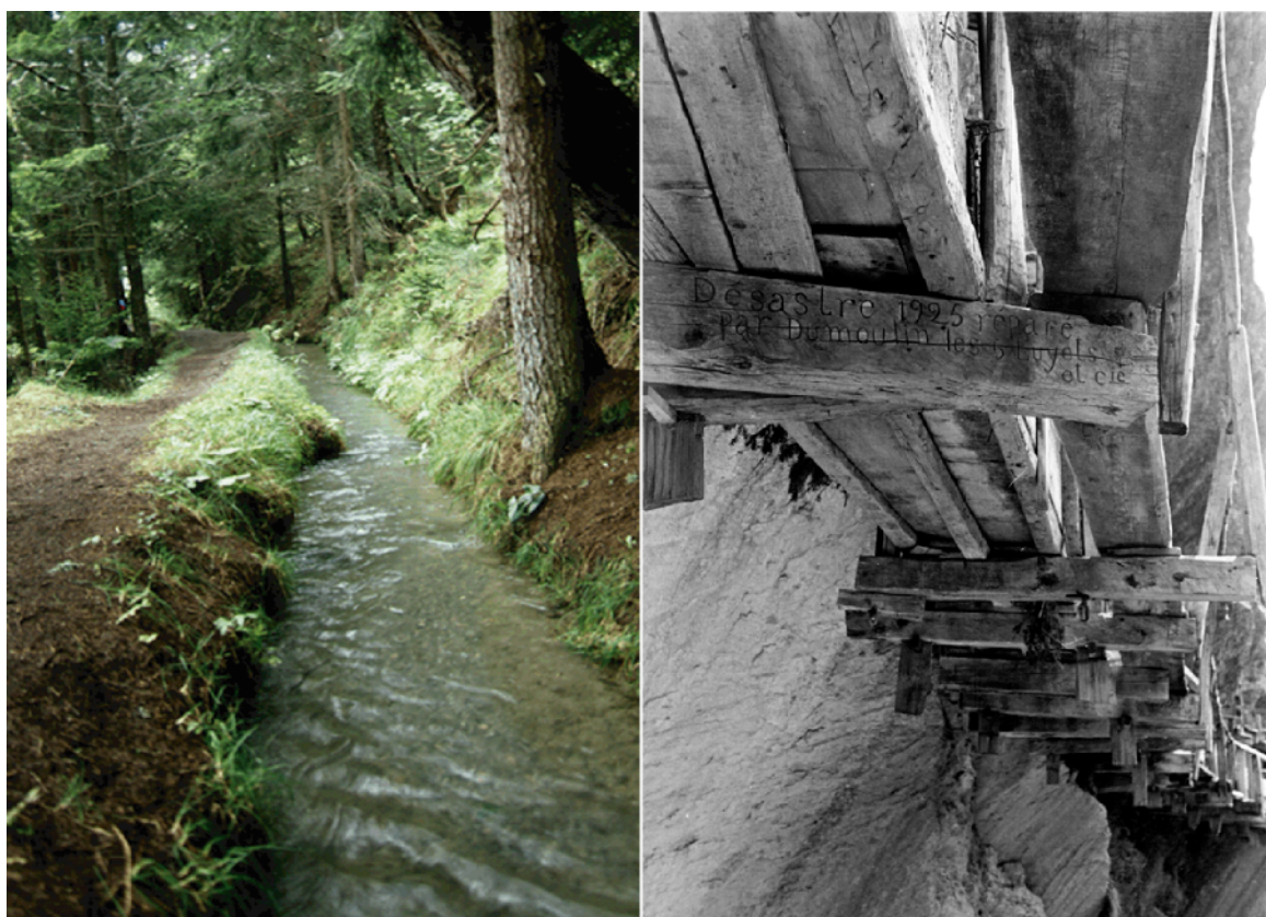
Figure 2 Channel cut into the valley side, the Bisce of Ayent (left), and wood channel, the former Bisce of Savièse (right).
