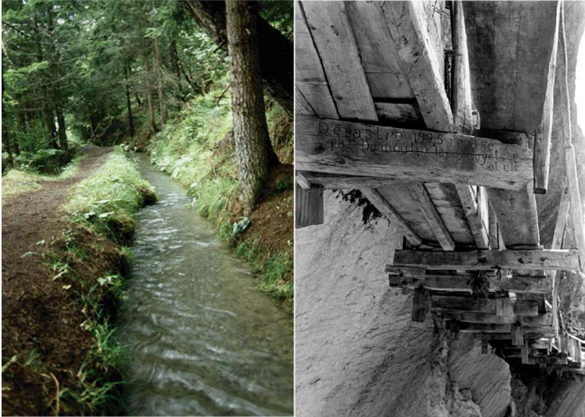
Figure 2 Channel cut into the valley side, the Bisse of Ayent (left), and wood channel, the former Bisse of Savièse (right).
